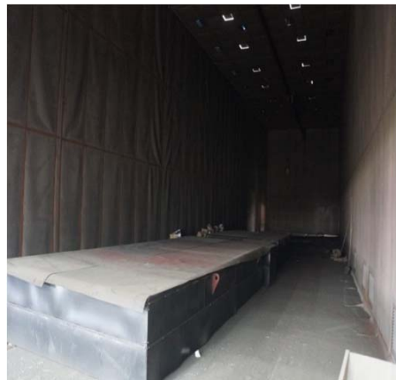
Painting Shop (8.5*9.5*35 meter)
